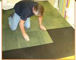
The 50m<sup>2</sup> of InstaLay was simply loose laid without the need for time consuming sub-floor preparations. The release film was then peeled back in stages and the carpet tiles positioned onto the low grab adhesive membrane and pressed into place.
