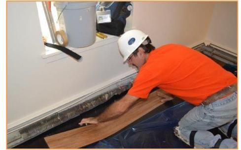
Completed in 2016, this installation at Marshall Field Garden Apartments in Chicago is, to date, the largest ever project to use InstaLay, the self-adhesive acoustic flooring installation system.
