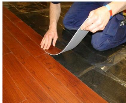
15. When a suitably large section has been fitted, it should be rolled at a 45° angle to the direction of the LVTs using a roller (roller weight of 45kg / 100lbs). Repeat this process for all additional sections until the entire floor has been fitted.
