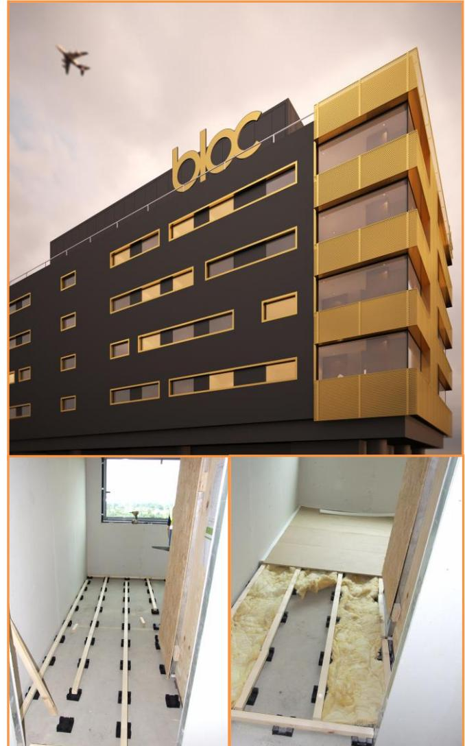
To comply with stringent fire safety requirements, fire resistant Intubatts were also installed in the floor void at room thresholds and corridor fire doors to help prevent fire spreading.
