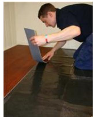
less half the normal time as no adhesive was required, eliminating any mess and open time. All that the fitter required to complete this quick and easy installation was a pencil, a tape measure and a sharp knife!
