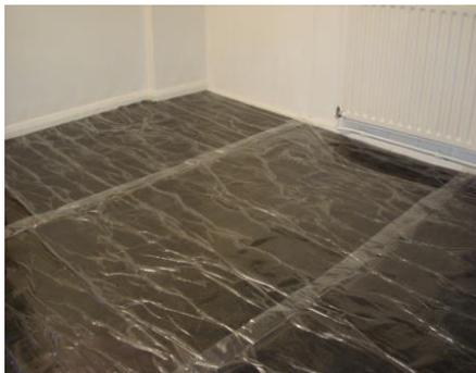
6. Cover the floor area to be fitted with InstaLay, leaving an expansion gap between the InstaLay and the perimeter wall and all fixed objects. Because this is a floating floor installation, it is recommended that a minimum 3mm (1/8in) expansion gap be maintained between the InstaLay and the perimeter wall and all fixed objects. This is necessary, as the installation may expand and contract with changes in temperature.
