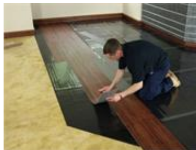
Setting out the LVT planks
