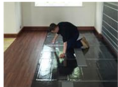
Laying the LVT planks
