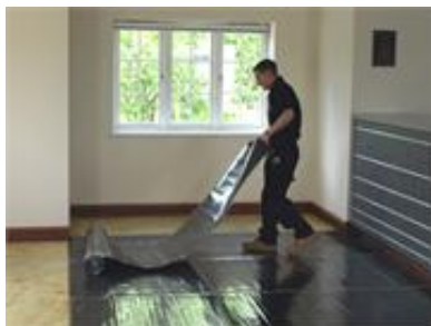
InstaLay being loose-laid
