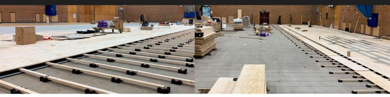
This challenge was met by designing and building a special level: this allowed the sports floor to maintain the sprung performance required for professional sports, with the ability to support the extra loads when required.
