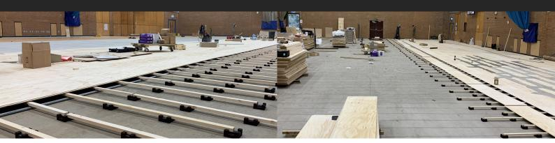
This challenge was met by designing and building a special level: this allowed the sports floor to maintain the sprung performance required for professional sports, with the ability to support the extra loads when required.
